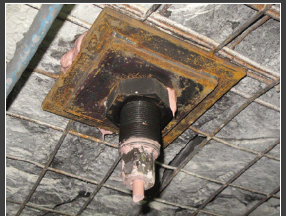
Grout telltale on completion of cable grouting
